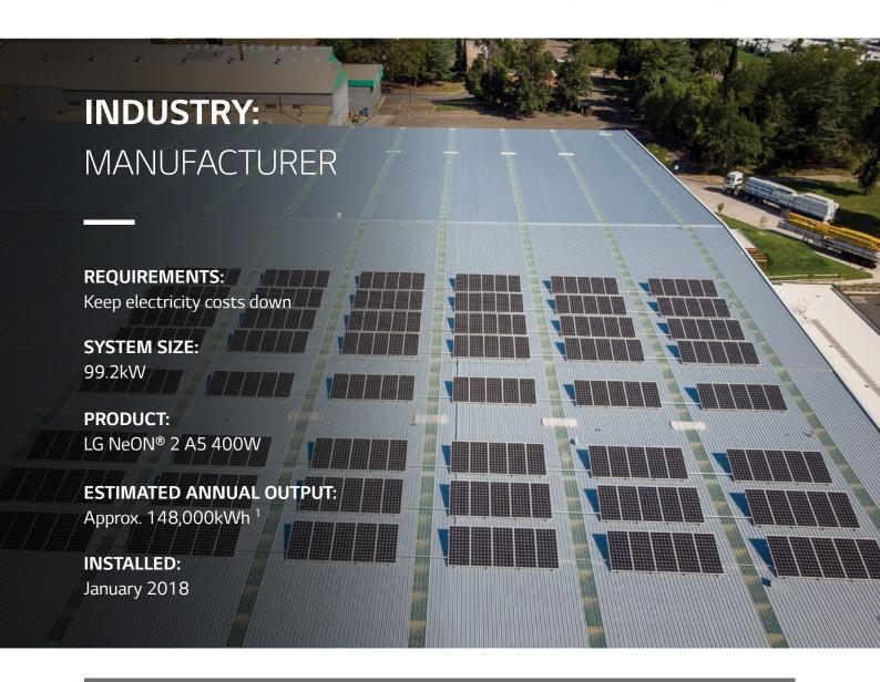
Design and install a high efficiency solar system to reduce power costs.
